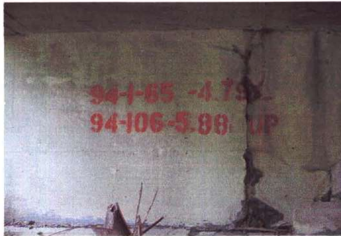
Br. No. Abutment No. 1
