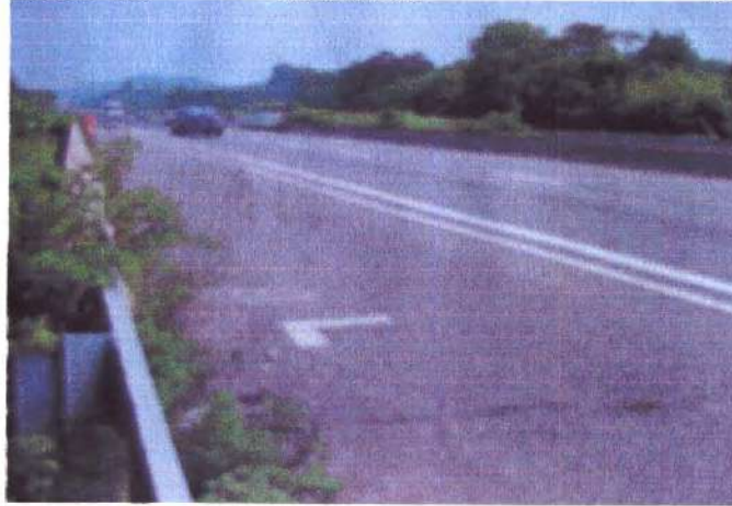
Across Top of Deck
