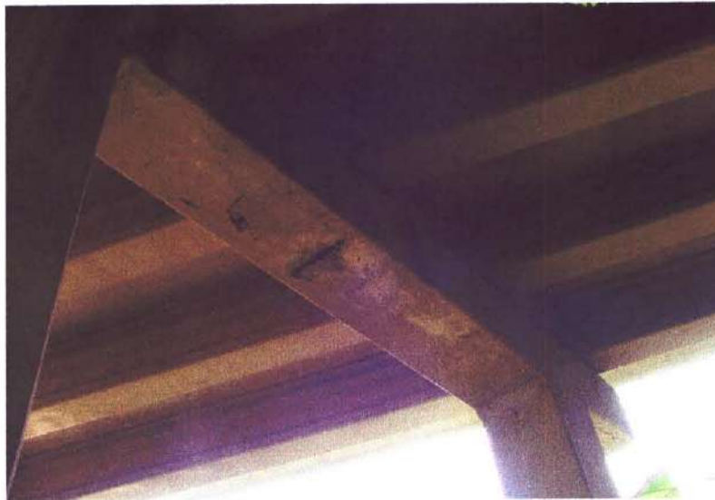
SPALL & REBAR, BOTTOM OF BENT CAP NO. 1
