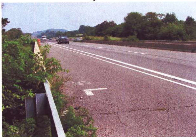
ACROSS TOP OF DECK
