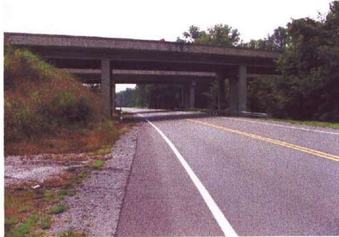
LOOKING BACK ON ROUTE- 94-106-5.88-UP
