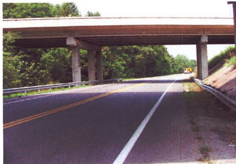
LOOKING AHEAD ON ROUTE (94-106-5.88 UP)
